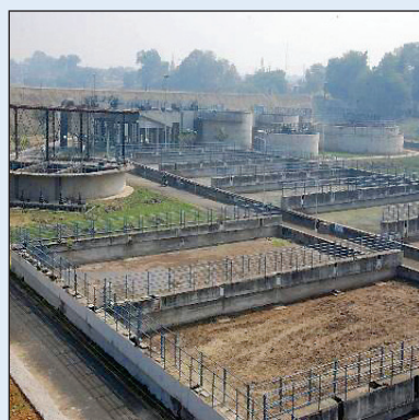
Treatment Plant, Varanasi
